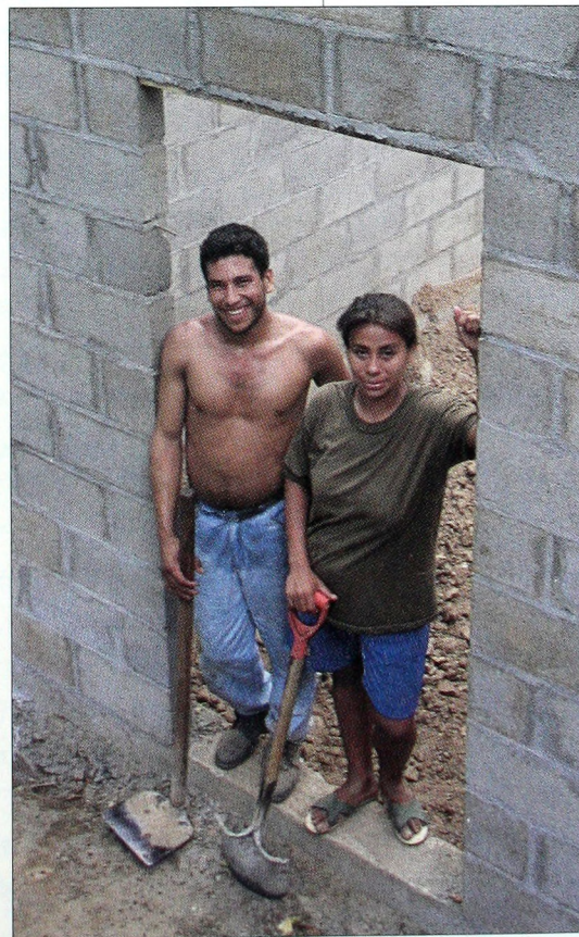
Raising the roof: Rafael and Blanca worked tirelessly on their home. "I think the children will be healthier in the new house," said Blanca.
